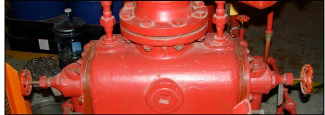
Turn on the pump by pushing the start button then close the two back pressure relief valves shown in the picture above. Close both right and left valves by turning them clockwise.
