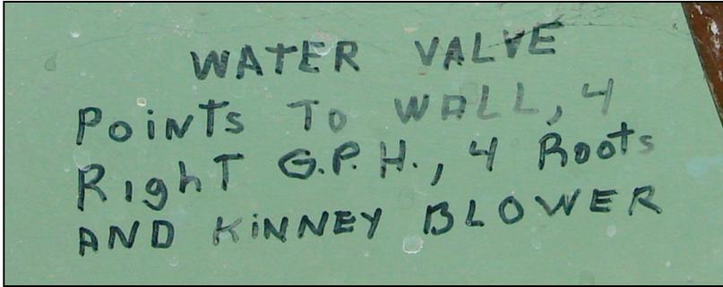
Read the writing on the wall. The faucet over the mop sink cold water valve handle gets pointed to the wall and that provides the flow of cooling water needed for the Kinney and Roots blower. Check the flow at the drain as stated on the previous page.
