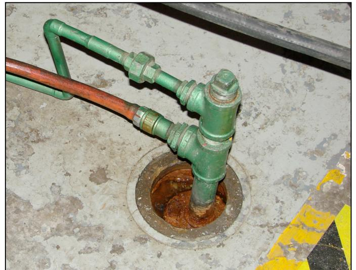
The hose hooks to the Kinney pump just above the pressure regulator and flows out into the drain in the floor. Remove the pipe plug in the drain assembly to see that water is really flowing from the two pipes then replace the pipe plug.
