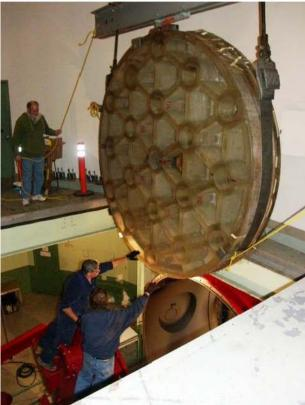
The mirror was lowered through the floor and the hook-shaped ends of the belly-band went over two permanent protruding beams in the tank.
