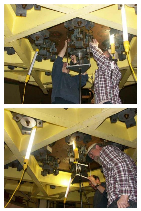
Meanwhile, the belly-band was carried by several people to the mirror, with the middle of the band at the mirror's North side. Two giant edge-arcs were hoisted over to the platform and bolted down.
