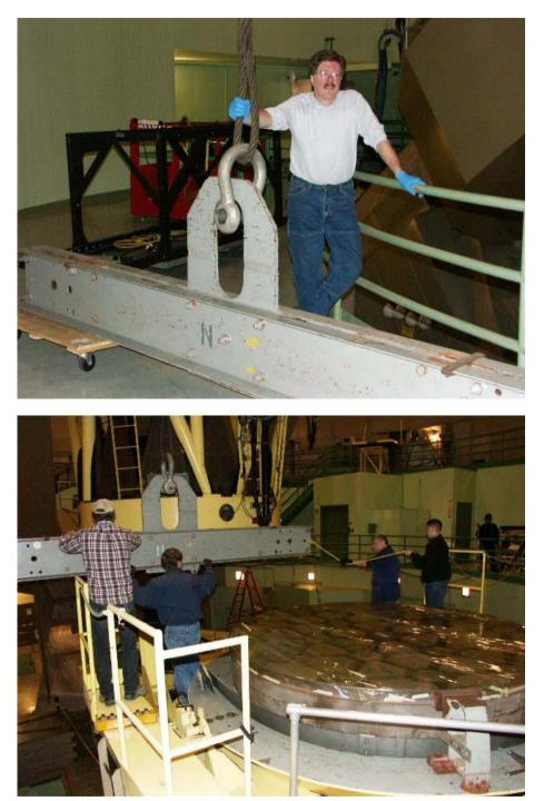
Two large jackscrews were fed through the I-beam and attached to the bellyband. The bellyband was supported by wooden blocks and also two extensions on the sides of the edge-arcs. One "earthquake bracket," just a C-shaped piece of metal, was attached to the I-beam and loosely gripped the mirror, and two more were attached to the belly-band at the sides.
