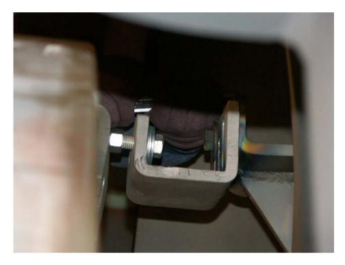
Another anchor was made by removing an "earthquake clamp" from one side and using the bolt on the belly-band to secure it to a fixed bracket in the tank.
